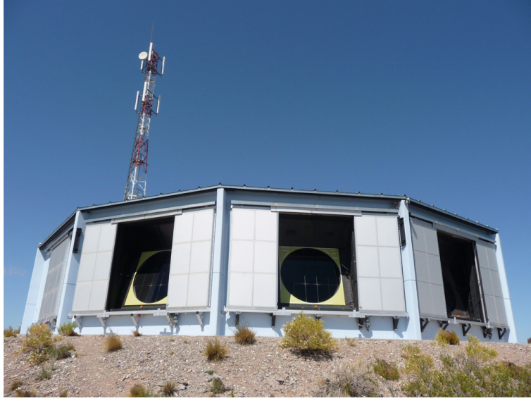
Figure 1.7: FD building at Los Leones during the day. Behind the building, there is a communication tower. The picture was taken during daytime; shutters were opened because of maintenance [15].
