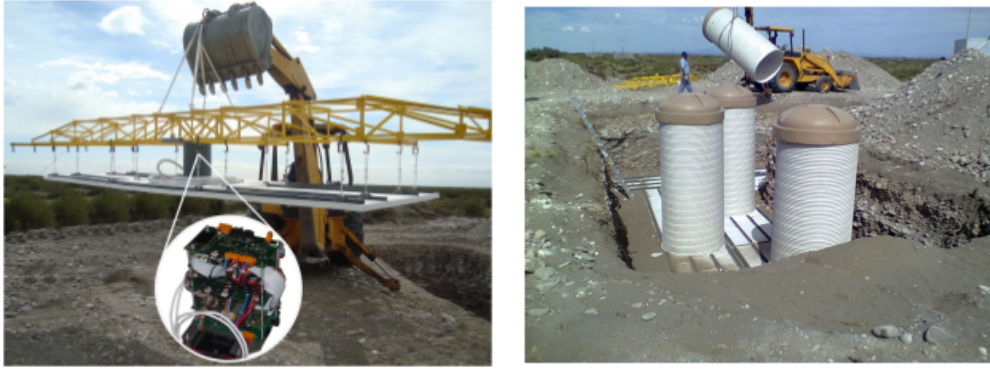
Figure 3.20: (Left) The deployment of the first MD module of the UC. The electronics kit, which is contained in a PVC casing, is shown in the inset [209]. (Right) Installation of an access tube during module deployment. The access tube is sealed to the module for water tightness [210].
