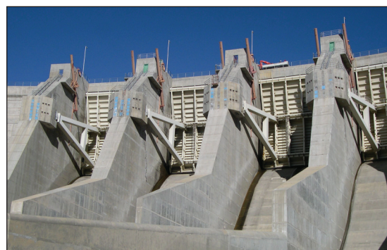
(b) View of the spillway and floodgates.
