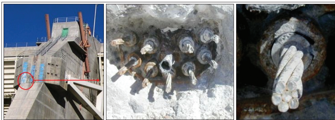
From left: (c) View of one of the piers studied. (d) Network of the fully grouted post-tensioned strands. (e) Detail of a strand.
