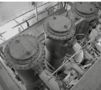
Central Nuclear Néstor Kirchner (ex Atucha II) Bombas de aceite
