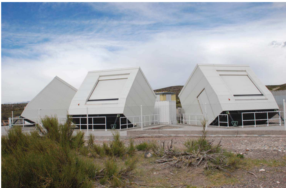
Figure 2.10: Photograph of HEAT in tilted mode with closed shutters [55].
