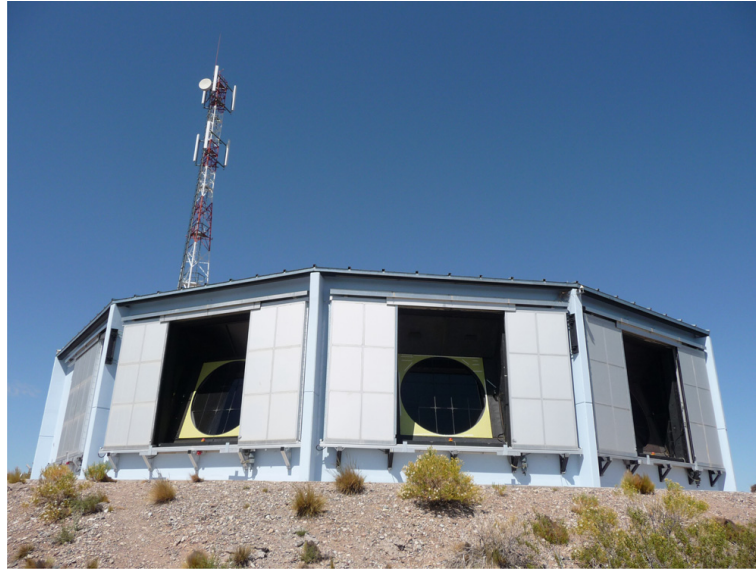
Figure 2.5: FD building at Los Leones during the day. Behind the building, there is a communication tower. The picture was taken during daytime; shutters were opened because of maintenance [17].
