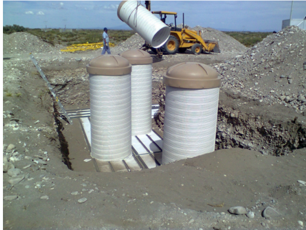
Figure 1.8: Installation of one of the 30\text{ m}^2 buried scintillation-based muon counters. These counters will directly measure the muonic component of EAS approximately at and below the energy of the spectrum's ankle. Picture from [9].
